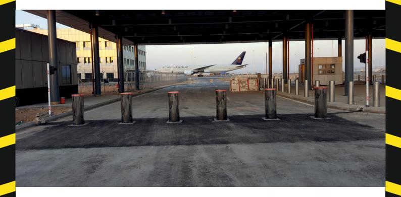
Panzer bollards are designed specially for place to high security with stainless steel body and hydraulic operation system.
